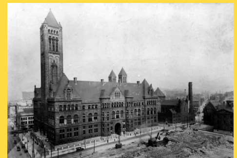
Third (Current) Courthouse under construction
